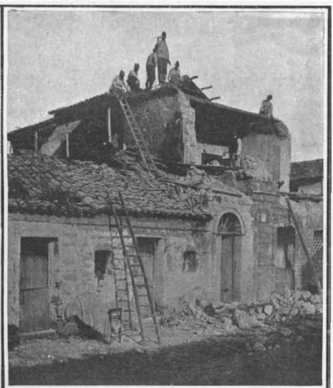
Soldiers razing walls in danger of falling.
